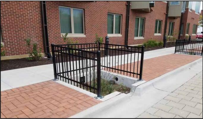
Figure 7. Tree well with Stormwater Management Feature
