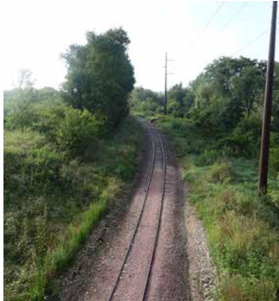
Veterans Memorial Parkway overpass
