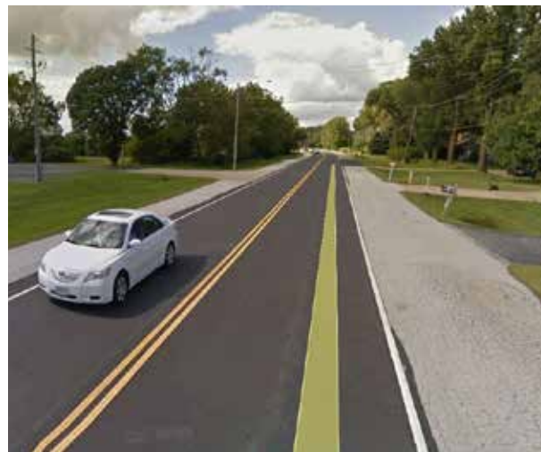
Paved shoulders on Northwest Boulevard
