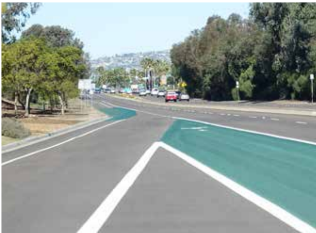
Buffered bike lane along a major arterial corridor in San Diego. Green paint is used to clarify bicycle traffic across access ramps effectively on even this limited access road.
