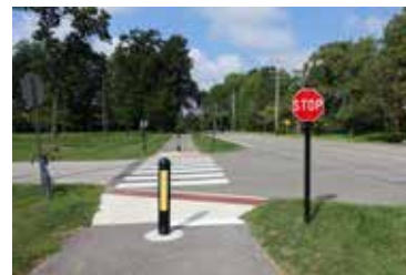
Sidepath with high visibility crosswalks and advisory trail crossing signs (Clayton Road, Saint Louis County, MO)
