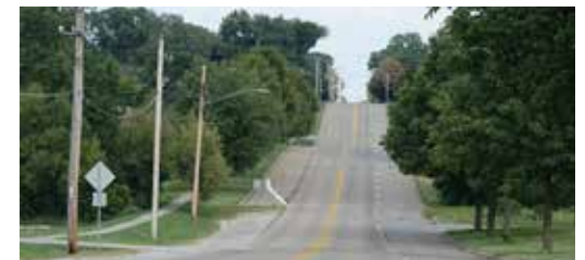
Low traffic, width, and relatively few interruptions may make a two-way protected bike lane feasible on Central Park Avenue's western leg.
