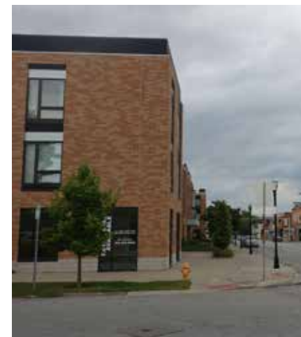
An emerging urban district like Hilltop becomes both a destination and point of origin in the network. Addressing issues in this area like offset intersections helps fulfill the directness and safety principles.
