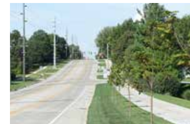
Tanglefoot Lane in Bettendorf offers both a sidepath and bike lanes in a complete street.
