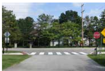
Sidepath with high visibility crosswalks and advisory trail crossing signs (Clayton Road, Saint Louis County, MO)
