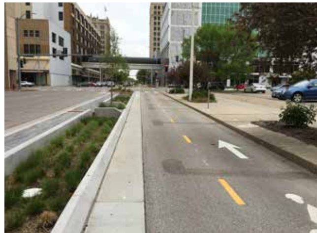
Top: One-way parking protected bike lane (Venice Blvd in Los Angeles' Mar Vista neighborhood) Above: Two-way protected bike lane with planter separation in Lincoln, NE.
