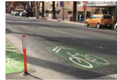
Enhanced sharrow with symbol in green box to increase visibility.
