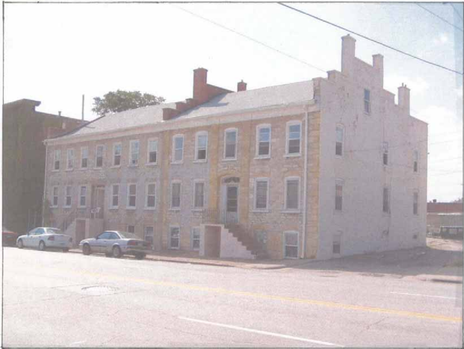
The West Third Street Historic District's greatest strength is its incredible variety of architectural styles. Among them is Hiller Row, 310-314 Gaines Street. The row of townhouses was constructed by John Miller, an immigrant stonemason from Württemberg, Germany. The row was constructed in three parts with the oldest section dating from 1852 with further additions in 1856 and 1859.
