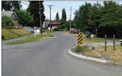
Chicanes create one-lane yield conditions. They can be used on both sides to deflect driver paths and further reduce speeds, though streets that are naturally narrow may not need this treatment.
