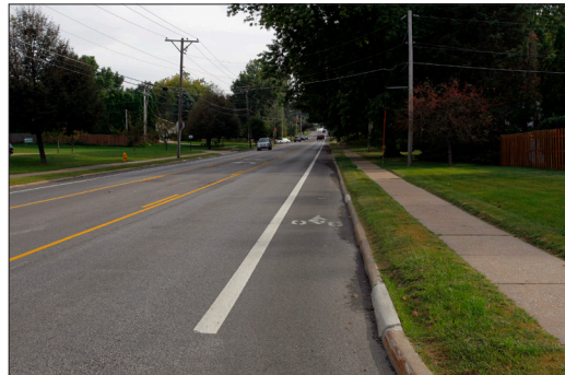
Existing on-street bicycle lanes on Jersey Ridge Road.
