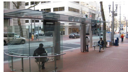
Bus shelters along the Portland, Oregon, Transit Mall offer seating, real-time information and rain guards.
