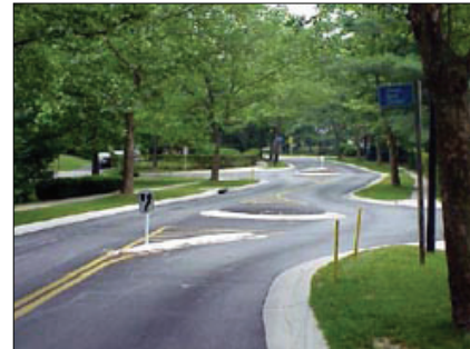
Roundabouts (above) and mini-roundabouts (below). Mini-roundabouts do not have the same traffic operations concerns as a larger roundabout, but given their smaller footprint are appropriate primarily on local, low-volume streets only.
