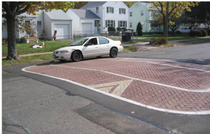
Speed tables are usually preferable to speed humps in that they are more accommodating to delivery and emergency vehicles, yet they also provide a cue to use lower speeds.
