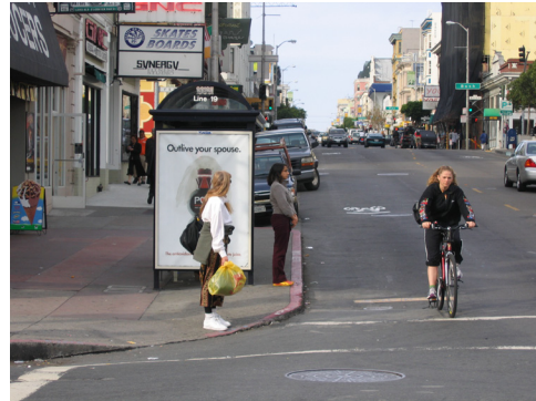
Bus bulbouts prevent delay caused when buses need to merge back into traffic after a stop.
