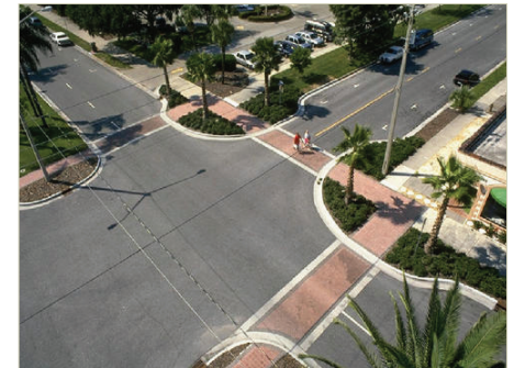
Bulbouts help to define parking areas as separate from drive lane areas (top) and, when used at intersections, shorten distances that pedestrians must cross (bottom).
