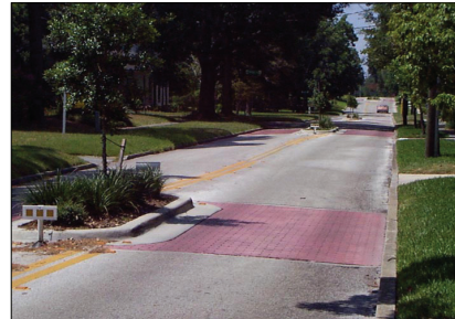
Median islands can be used to narrow travel lanes. Lanes remain passable but prompt drivers to move more slowly around the median.
