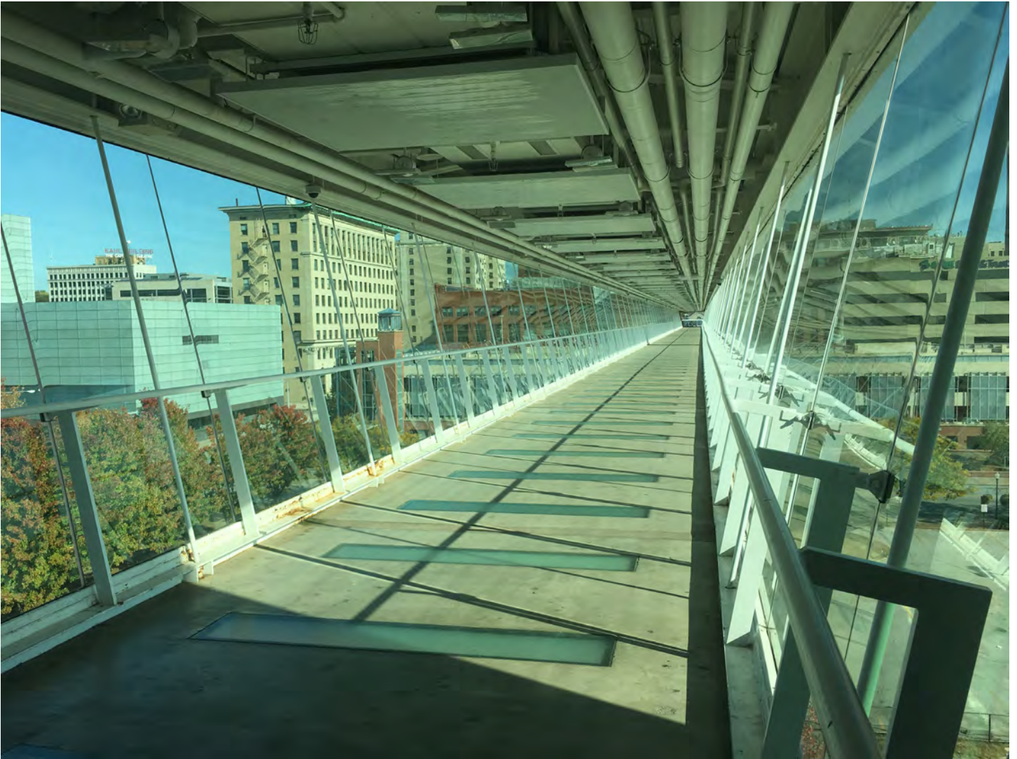
The Skybridge connects the Redstone Parking Ramp and the Riverfront, creating a dynamic observation point to see downtown and the Mississippi River.
