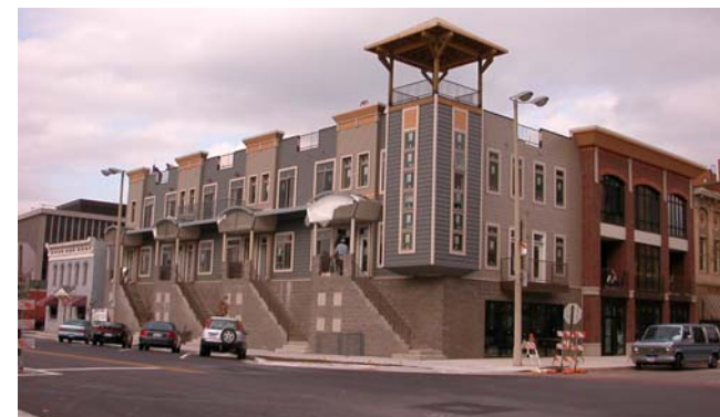
Construction of the Clipper Condos, Rock Island
