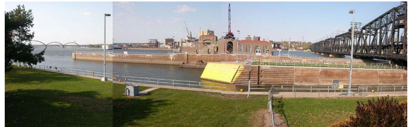
Lock and Dam 15
