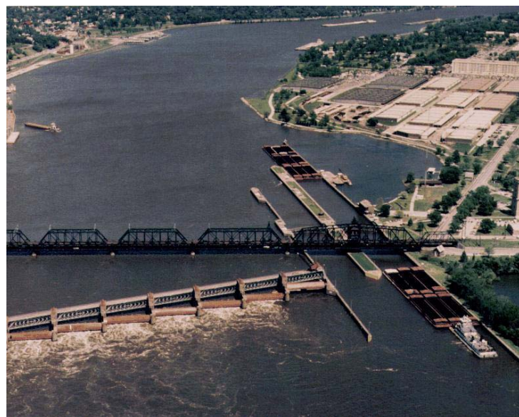
Lock and Dam 15
