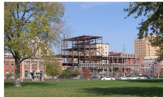
Construction of the Figge Art Museum, Davenport
