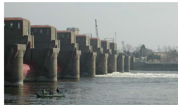
Lock and Dam 15
