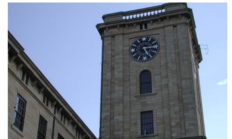
Arsenal Island Clock Tower
