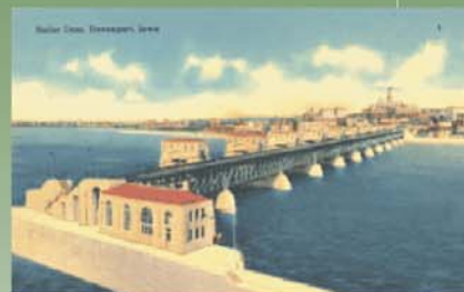
Roller Dam, Davenport
