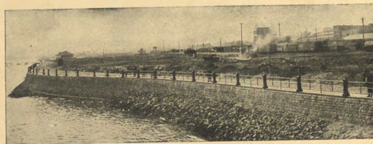
THE SEA WALL FIRST CONSTRUCTION WORK IN RECLAMATION OF DAVENPORT LEVEE
